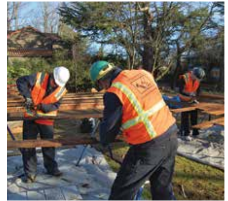
Credit: Lovett Deconstruction
