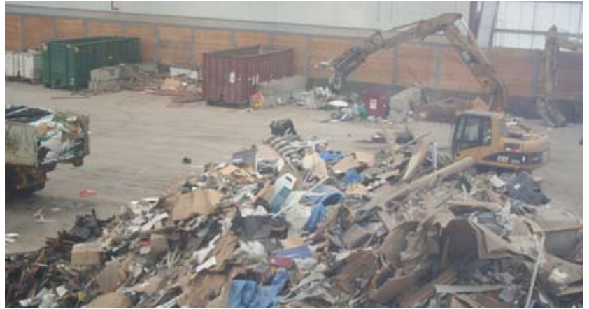
Waste Management Hillsboro Landfill Dry Waste Material Recovery Facility.
